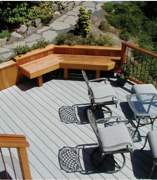
Left: Build deck at least 12 feet wide. Photo courtesy of Decking Northwest
